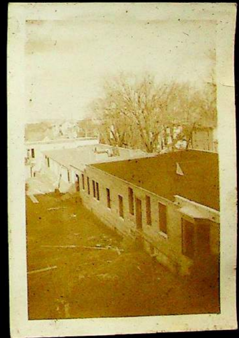
JUNIOR COLLEGE BUILDING UNDER CONSTRUCTION
