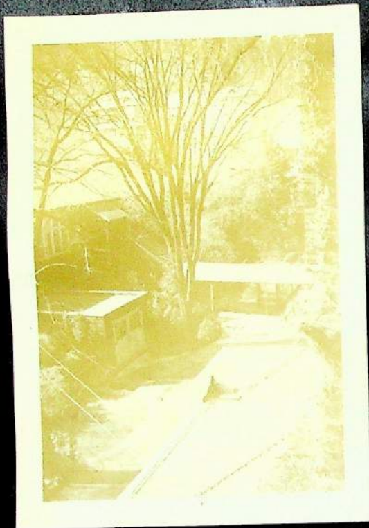
Front drive from Fire escape
