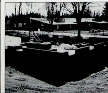
A step further: the Middle School foundation is laid.
