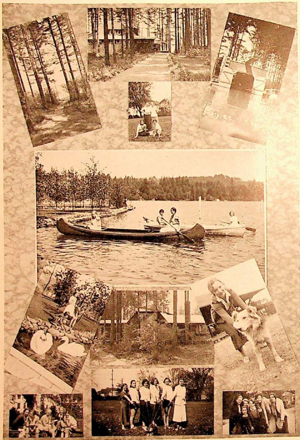
VIEWS AT EVERGLADE, OUR LAKE OSWEGO HOME
